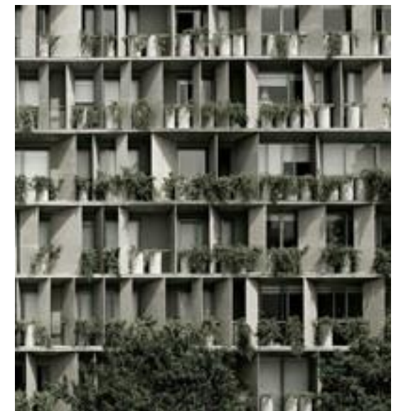
- UN Park apartments
